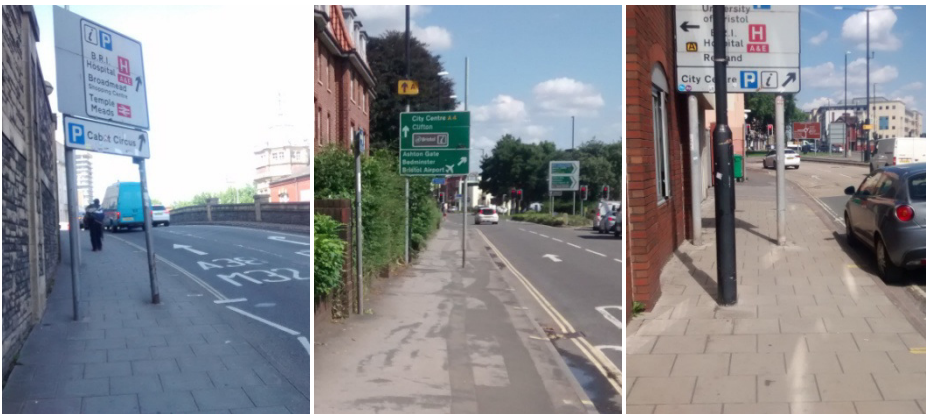
Obstructive road signs
